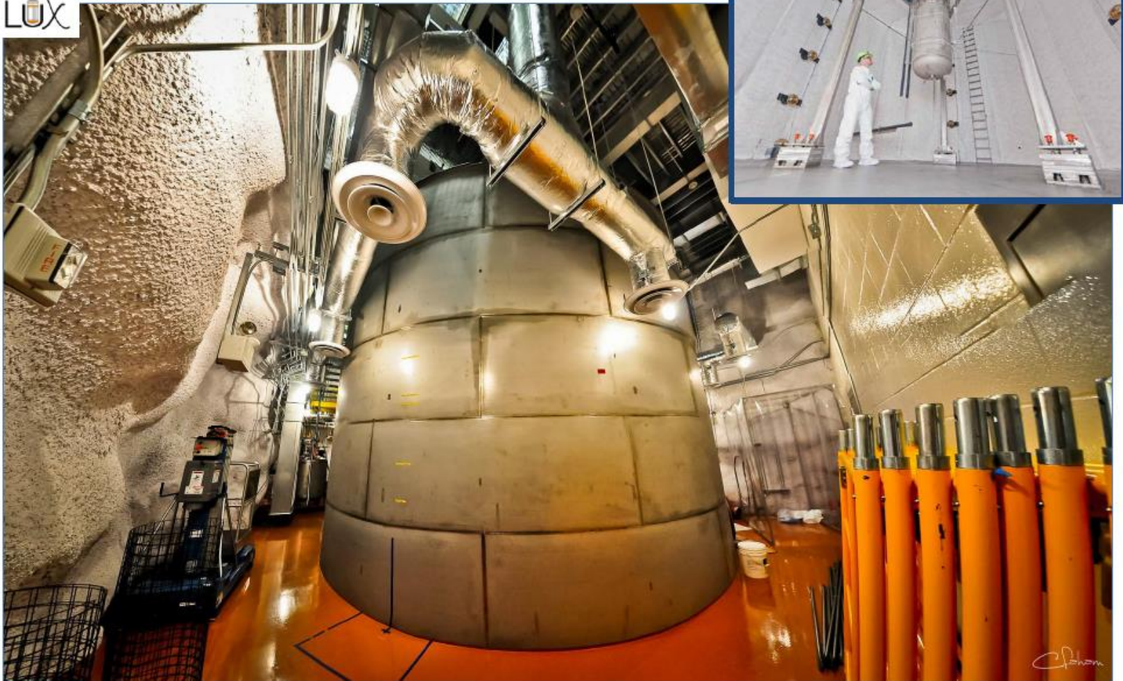
The 8-m diameter LUX water tank (to contain LZ), Davis Campus, 4850-ft u/g level, Sanford Underground Research Facility
